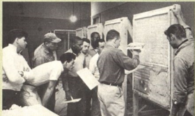
Job trainees in New York learn how to plaster a wall in 1965
